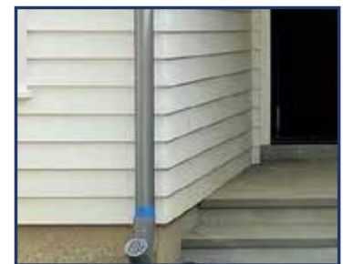
5/8 x 8 Beveled Siding, Smooth Face with Mitered Corners
