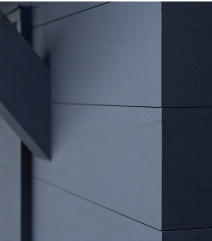
NO NEED TO PRE-DRILL OR PRIME ENDS OR FIELD CUTS
