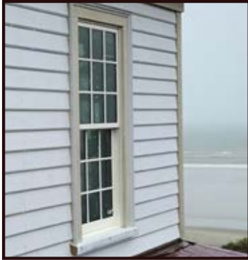
Custom Siding, Casing, and Sills Private Residence Kiawah Island, SC
