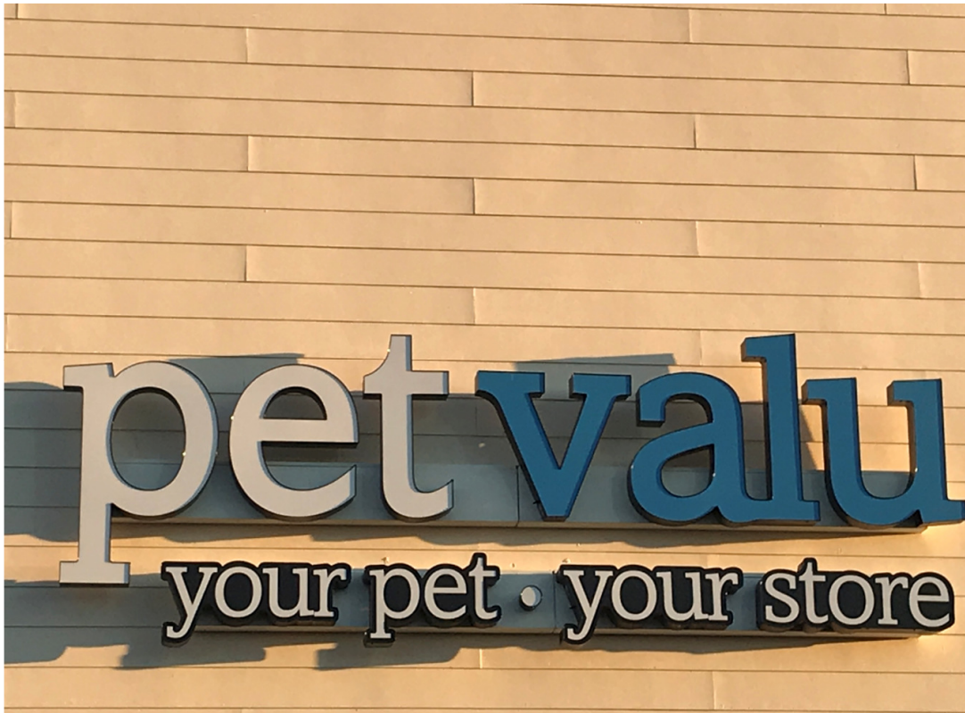
Pictured: The result of water infiltration on the ends of FC siding boards
